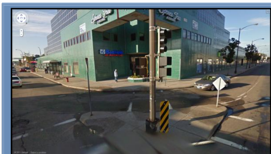
Figure 1: Wide corner radius and pedestrian island on the corner of University and Snelling by the Spruce Tree Centre
