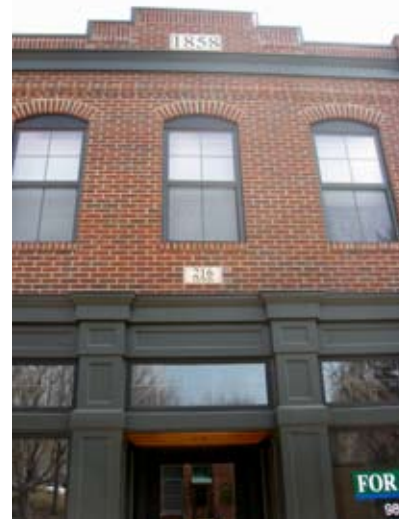
Figure 2. Built in 1858, Watertown used funding from the Small Cities Development Grant to renovate the exterior of this building, using design standards to preserve historical character. 5 Photos by Leah Roth-Howe.
