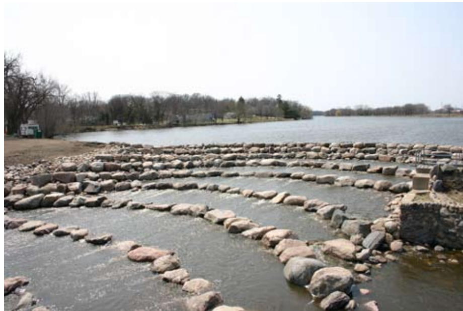
Figure 1. Hutchinson fish ladder. Photo courtesy of the City of Hutchinson.
