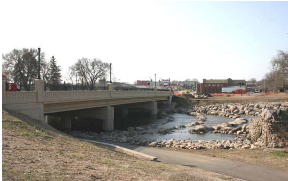
Figure 2. View of new bridge, fish ladder, the Luce Line trail and downtown Hutchinson. Photo courtesy of the City of Hutchinson.
