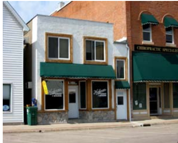
Figure 1. Renovated buildings along Lewis Avenue above illustrate how architectural design enhances uniformity as well as the aesthetic quality of downtown. The brick building on the right was built in the 1800s, while the two on the left are recent additions to Lewis Avenue. 4
