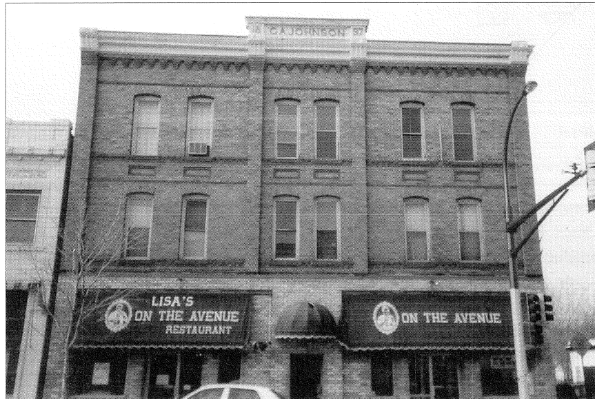
One example of a building facade worth improving.
