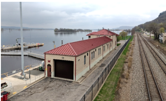
Figure 2.11: Lock and Dam No. 4. Top: View of a roller gate from the top. Middle: Side view of Lock and Dam No. 4. Bottom: Control building for Lock and Dam No. 4. (source: Maddie Loeffler)
